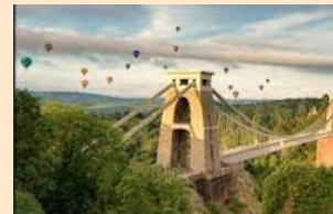
Clifton Suspension Bridge - Bristol
